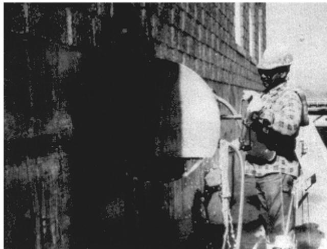
**Figure 5-3. Diamond-blade saw**
