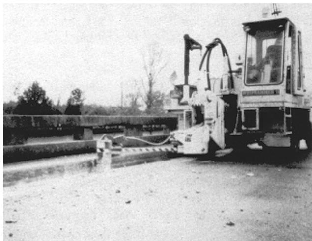
Figure 5-8. Spring-action hammer (mechanical sledgehammer)
